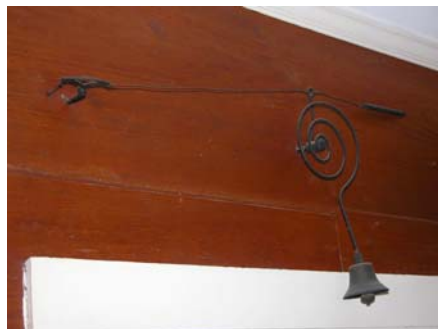
1.26 Service bell in former winter kitchen of Col. Means mansion, July 6, 2008.
