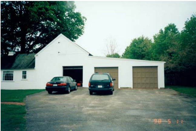
1.35 The former shed hid the pleasing form of the small barn, and created a sea of asphalt that was good for sports, but bad for the eye. Photographed May 11, 1998.
