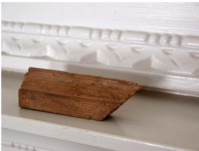
1.23 Scrap of ogee molding, with pencil marks, found in wall of parlor during sill repairs by Tony Hall on September 23, 2002.
