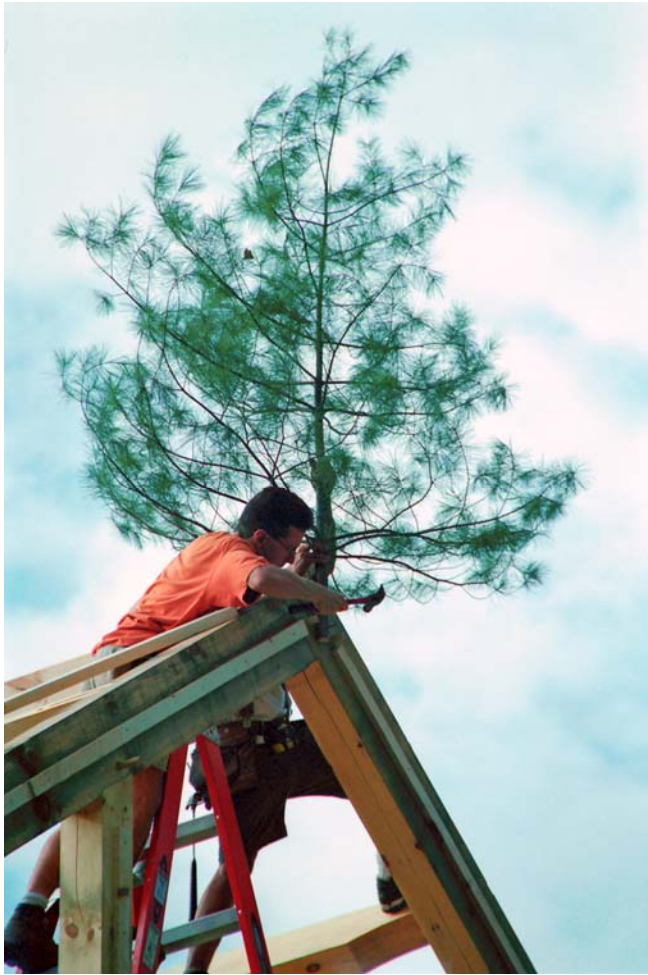
1.37 Bill Veillette nailing a bough of white pine to the peak of the barn frame, September 10, 2001. It is tradition to consecrate a frame with a bough from the species of tree from which it was cut. The frame of the big barn at the Col. Robert Means mansion is mostly eastern white pine for the posts and beams, and white oak for the braces. Photograph by Tracy Veillette.
