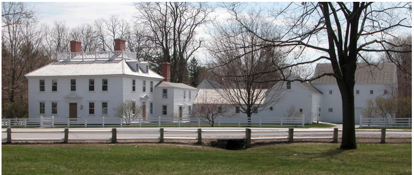
1.8 Col. Robert Means mansion, Amherst, N.H., April 22, 2004, showing its main block, ell, back house, small barn, and big barn. The house was rehabilitated by William and Tracy Veillette between March 2001 and August 2003.
