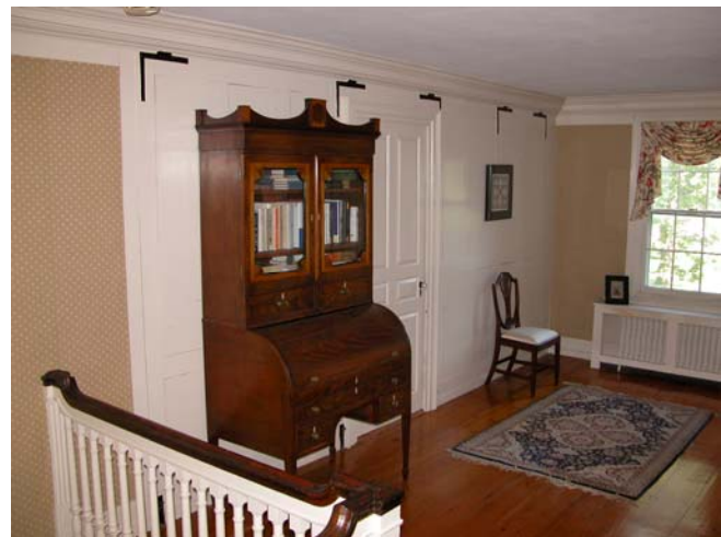
1.19 Paneled wall in center hall of the Col. Robert Means mansion, August 23, 2008. The wall is hinged so that it may be lifted and hooked to the ceiling to create a ballroom for dancing.
