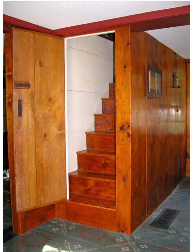
1.27 Staircase in summer kitchen in ell of Col. Robert Means mansion, August 24, 2008. Such narrow, steep, boxed-in stairs are becoming rare and should be preserved.
