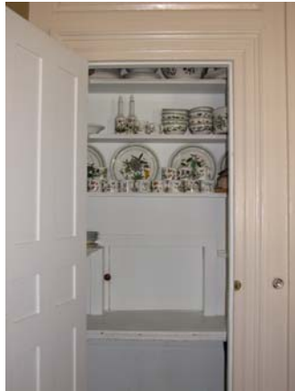
1.25 The food pass-through was a practical feature promoted by Andrew Downing in 1842. Abby Means installed hers in 1846.
