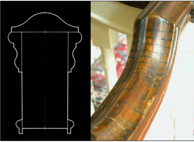
1.17 Profiles of moldings and construction detail of handrail on central staircase of Col. Robert Means mansion, July 19, 2008.
