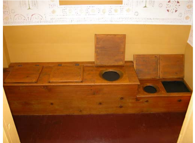
1.33 The privy, August 23, 2008. Other than conservation work, the privy has not changed since its original installation.
